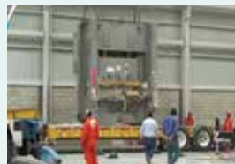
Onsite Installation Post-Relocation Services
