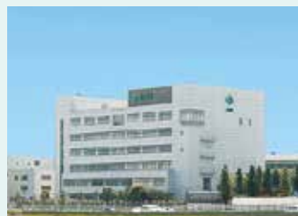
AIDA ENGINEERING, LTD. Site area: 184,000 m 2 Building area: 180,000 m 2
