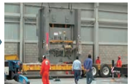
Onsite installation work. AIDA also continues to provide after-sales services after equipment is relocated.
