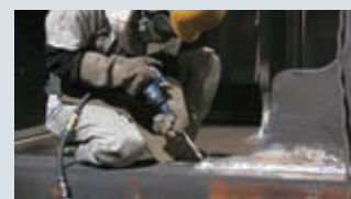
Hammer peening a weld to increase its fatigue strength
