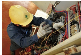
Work being performed by experienced press machine technicians
