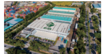
AIDA ENGINEERING (M) SDN. BHD. AIDA MANUFACTURING (ASIA) SDN. BHD. Site area: 72,000 m 2 Building area: 32,000 m 2
